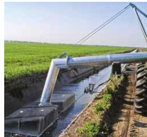
Individual solution: floating suction line
